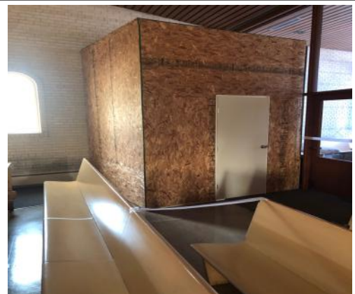
Designated protected work area for lift entrance into the Church
